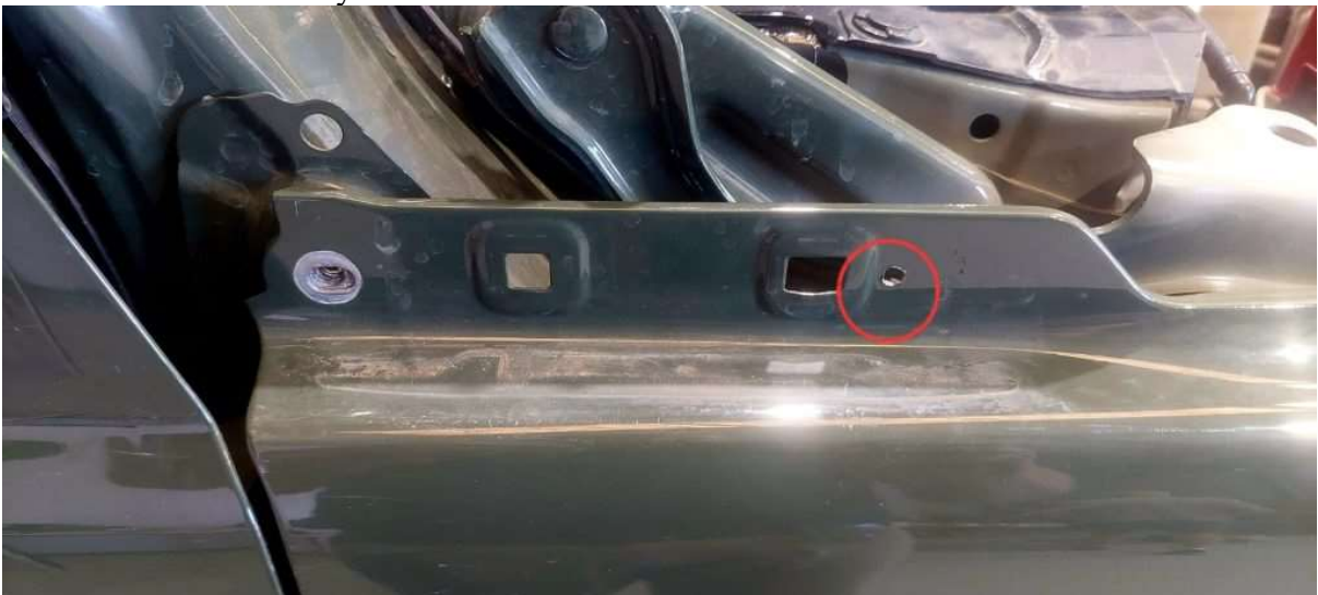
Suzuki Jimny Bravo Snorkel Installation Guide - Drill Hole in fender 3
